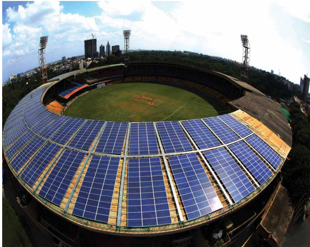
Solar panels fitted on top of the East Stand at KSCA's M. Chinnaswamy Stadium (above) along with power saving LED lighting (right)
