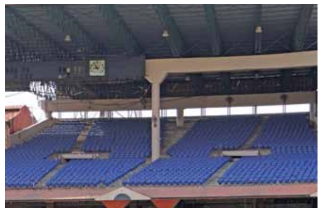
M. Chinnaswamy stadium Permanent seating
