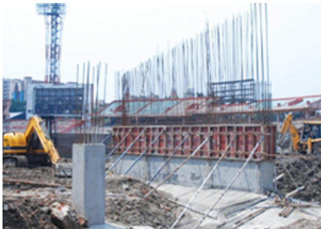
Reconstruction work in full swing at Eden Gardens, Kolkata
