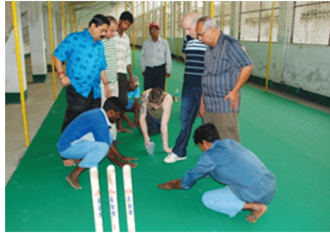
Indoor Academy surface being laid
