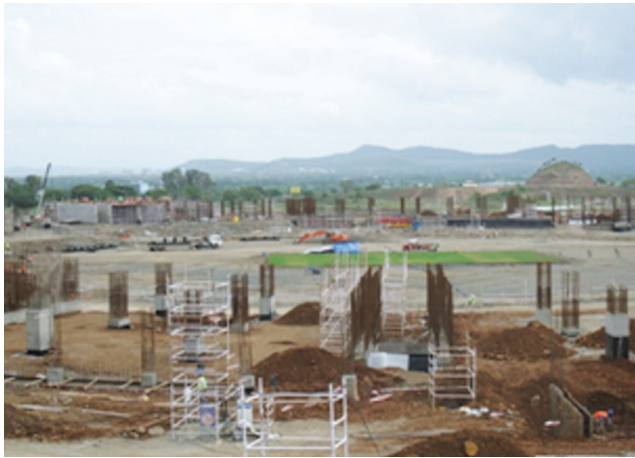
Work in progress for the stadium
