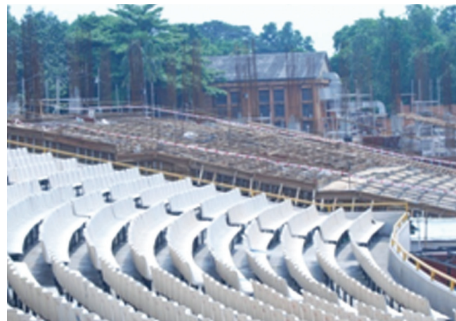
A completed section of the stadium
