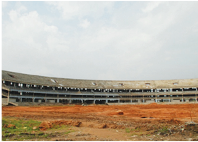
Stadium under construction
