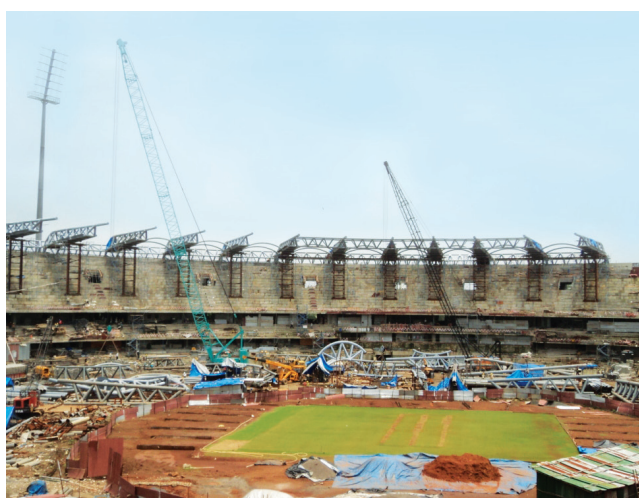
Construction in full swing
